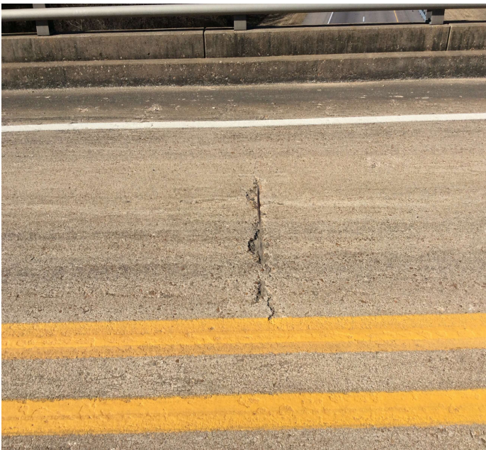
PHOTO 1 Description Typ. Delam, Cracking & Spalling W / Rebar Exposed in Spans 2 & 3. Rebar too close to Surface.
