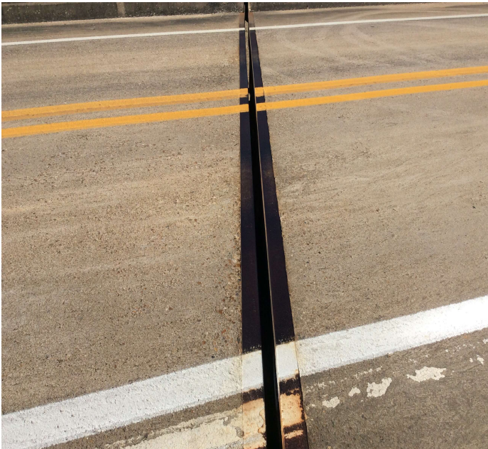
PHOTO 1 Description Joint Seal missing at Pier 3.
