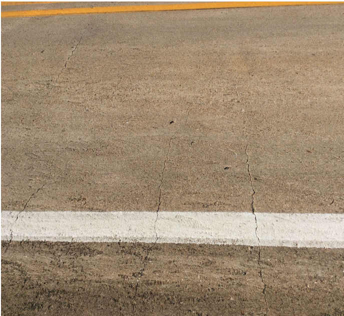
PHOTO 1 Description Typ. Cracking in Deck.
